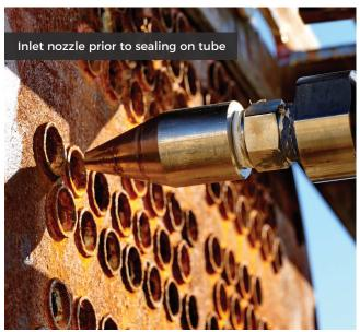
CONTROLLED-VOLUME PIGGING HAS REDUCED TURNAROUND TIMES BY UP TO 66% COMPARED TO FLEX LANCING AND OTHER CLEANING METHODS.
